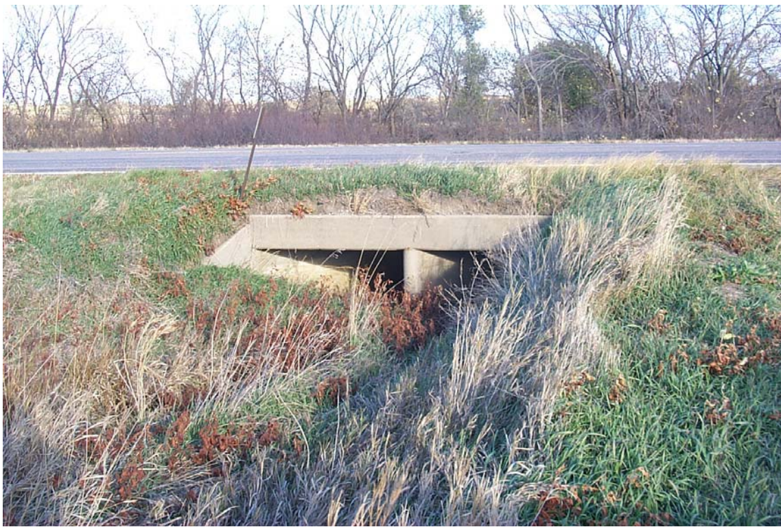
Figure 1. Low Fill Culverts
