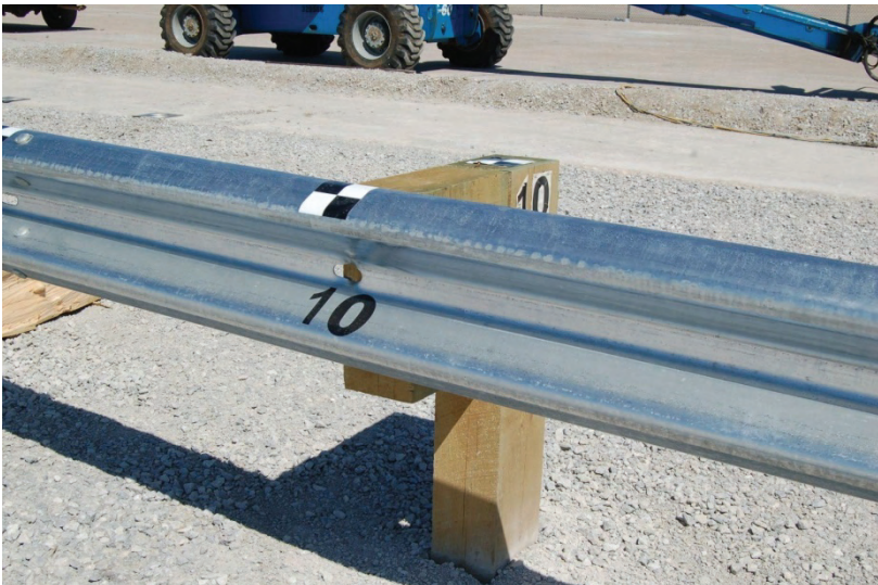
Figure 33. Post Nos. 8 through 10 Damage, Test No. MGSWP-1
