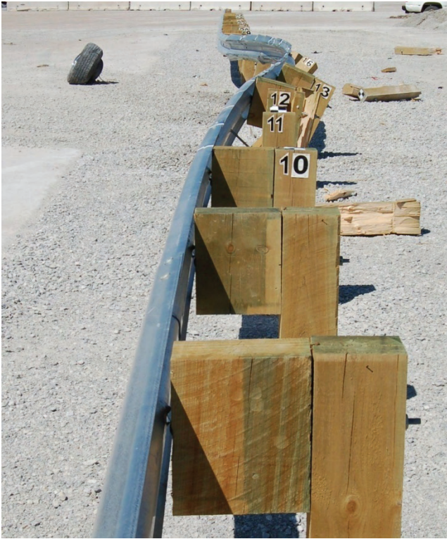
Figure 31. System Damage, Test No. MGSWP-1
