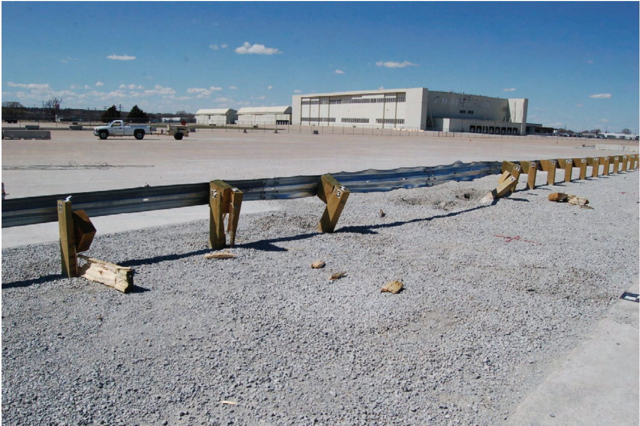
Figure 30. System Damage, Test No. MGSWP-1
