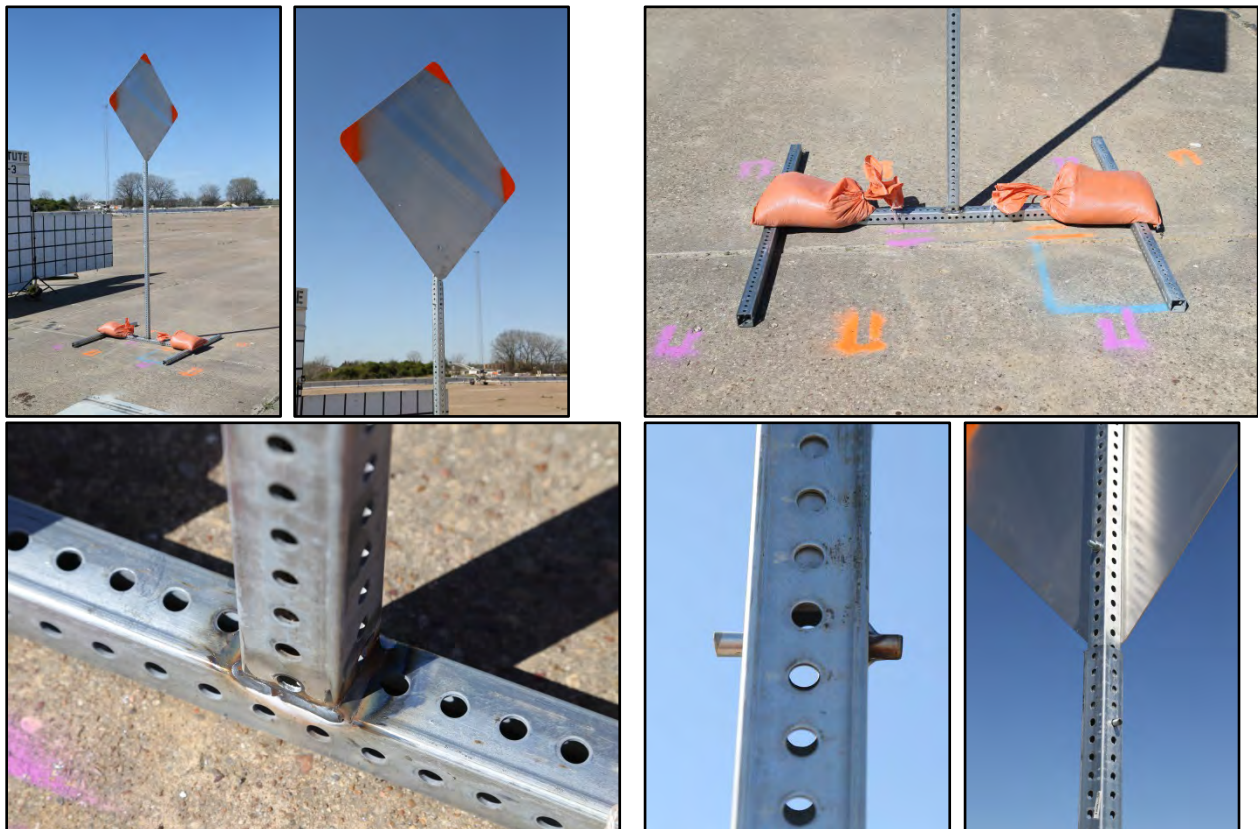
Figure 7.8. Option C Temporary Work Zone Sign Support Used for Test No. 490026-2-5.
