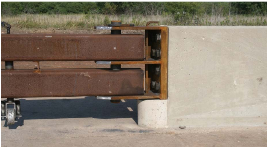
Figure 1.1. Emergency Opening System (EOS).
