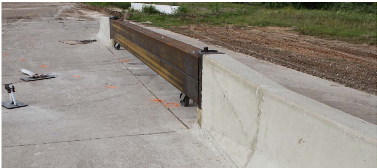
Figure 3.3. TxDOT Median Barrier Gate Installation before Testing.
