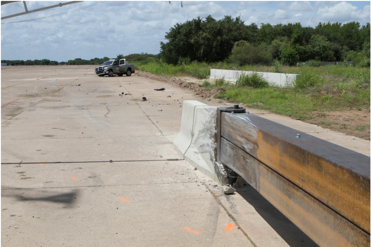
Figure 8.3. Position of Vehicle/Gate after Test No. 420020-8.
