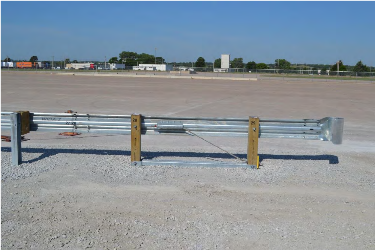
Figure 127. Test Installation Photographs, Test No. WIDA-2
