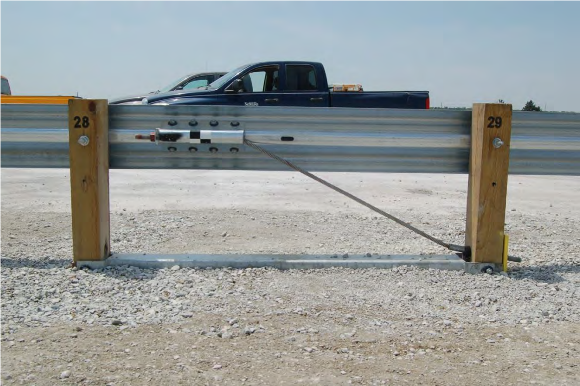
Figure 122. Test Installation Photographs, Test No. WIDA-1
