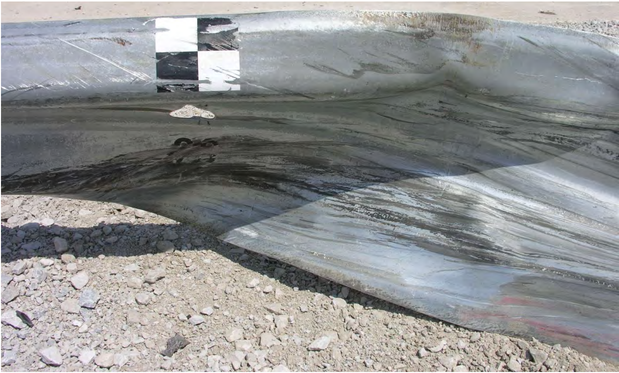
Figure 153. Rail Slot Tearing at Post Nos. 27 and 29, Test No. WIDA-2
