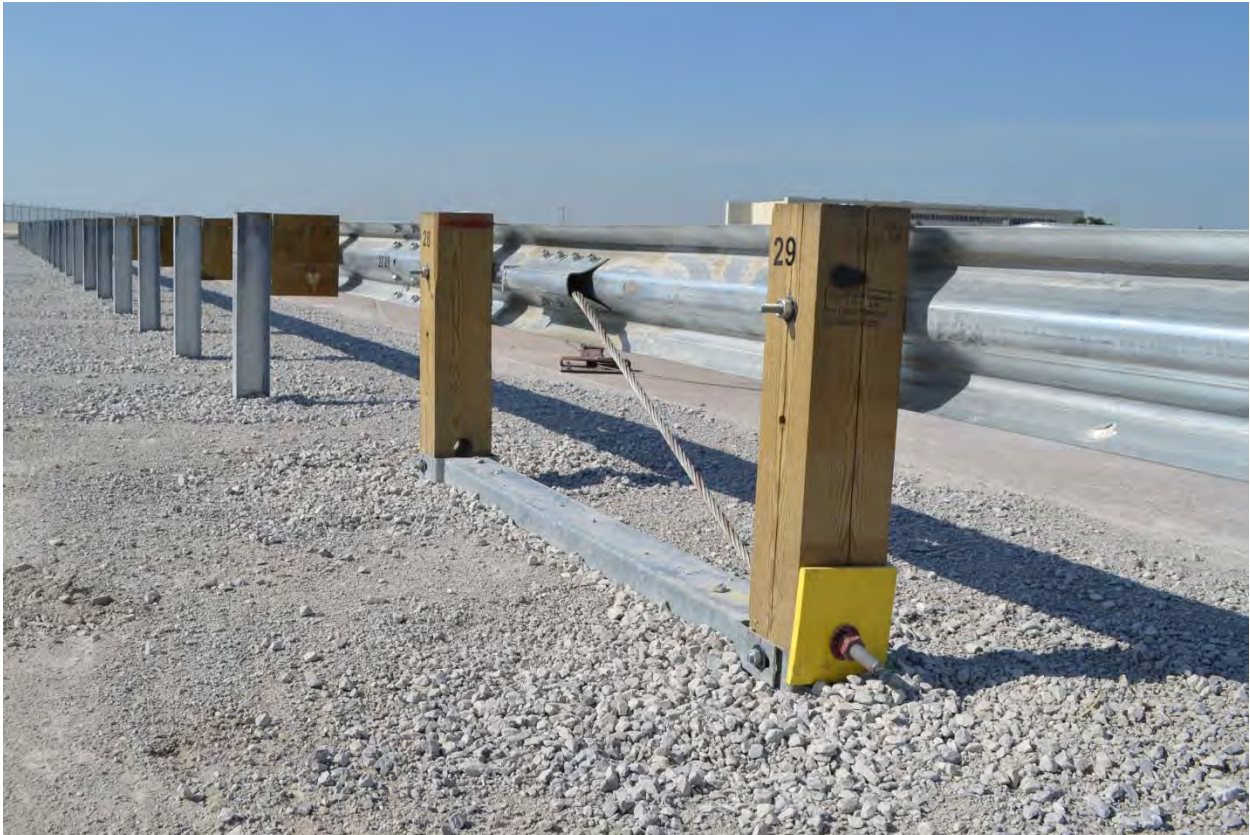
Figure 125. Test Installation Photographs, Test No. WIDA-2
