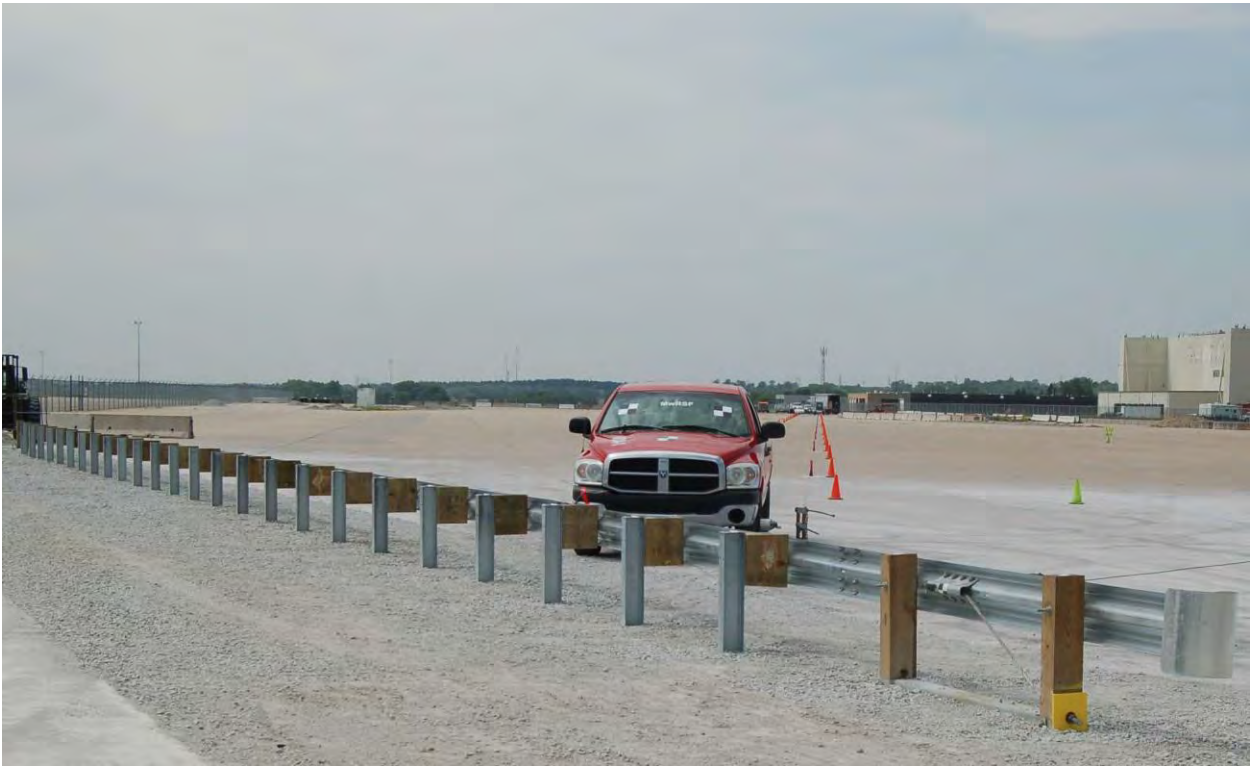
Figure 120. Test Installation Photographs, Test No. WIDA-1
