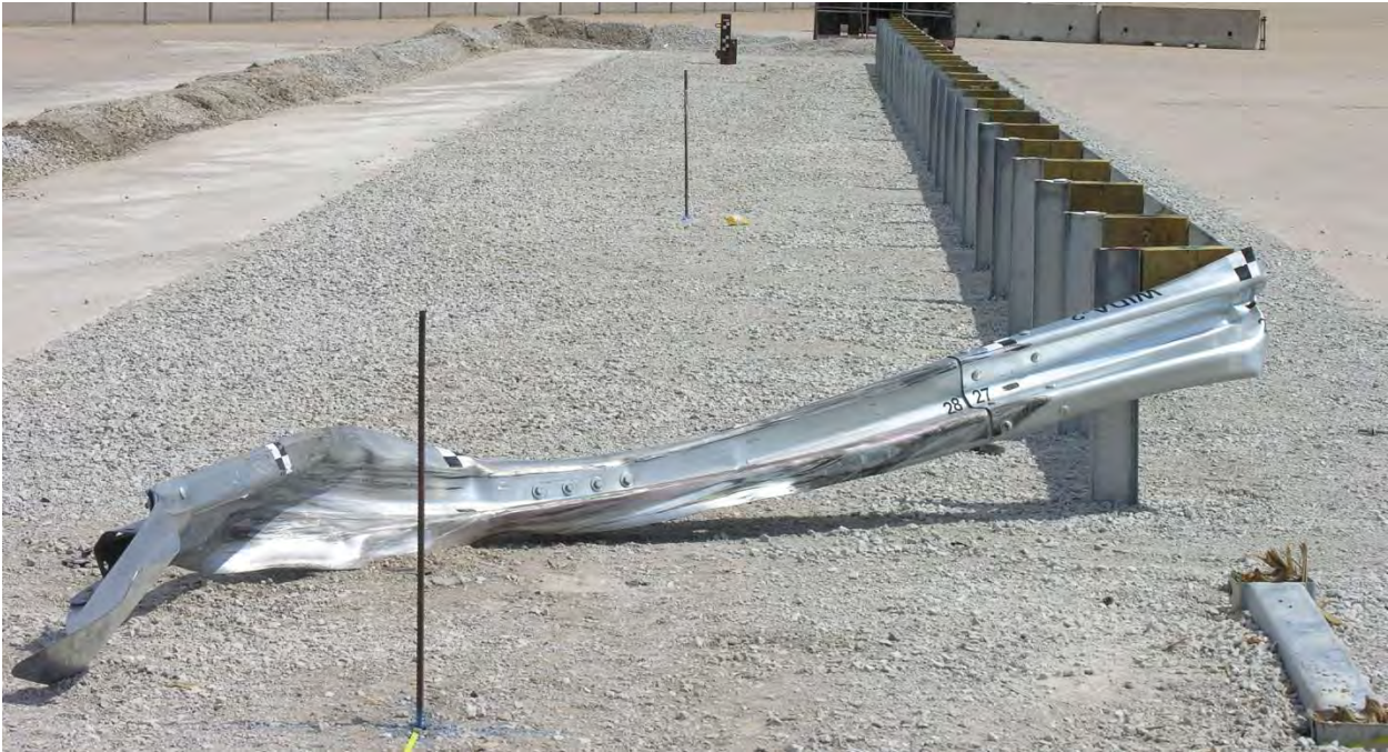
Figure 152. System Damage, Test No. WIDA-2
