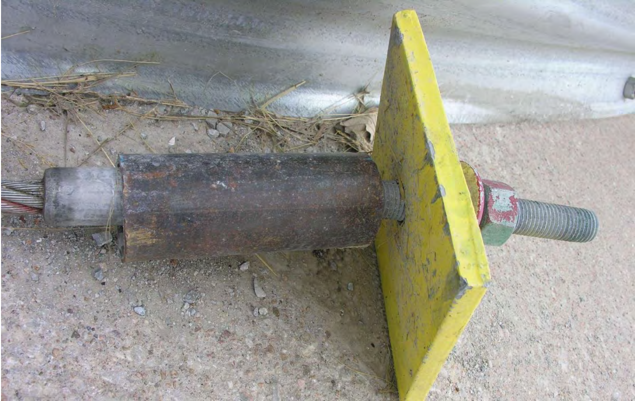
Figure 141. Anchor Cable Damage, Test No. WIDA-1
