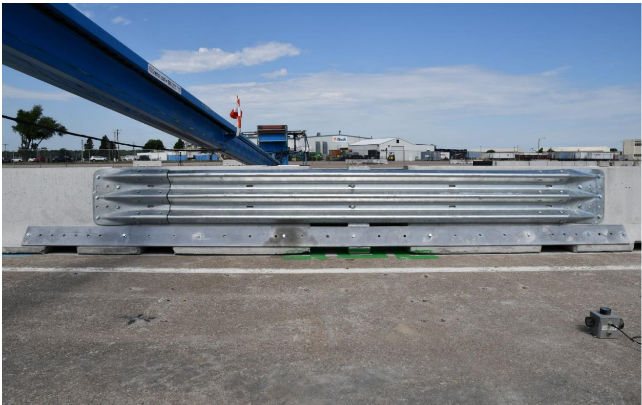
Figure 64. Test Installation Photographs, Test No. GSH-2
