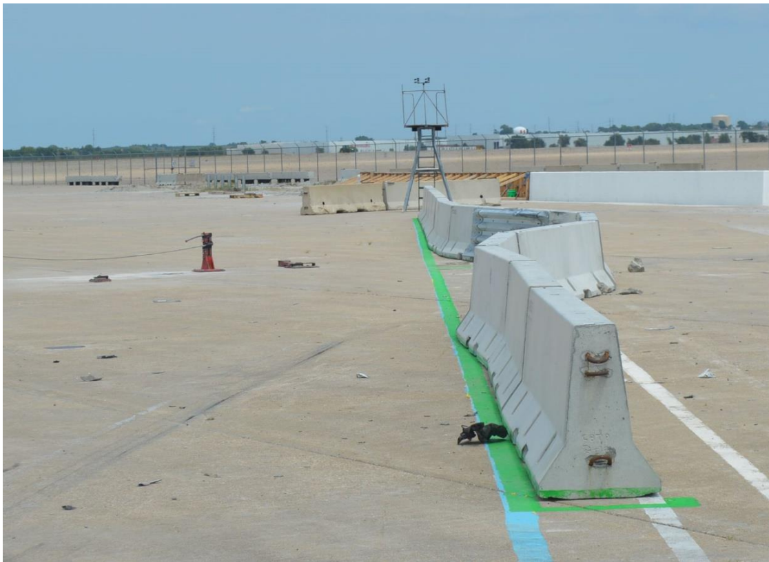
Figure 72. Overall System Damage, Test No. GSH-2
