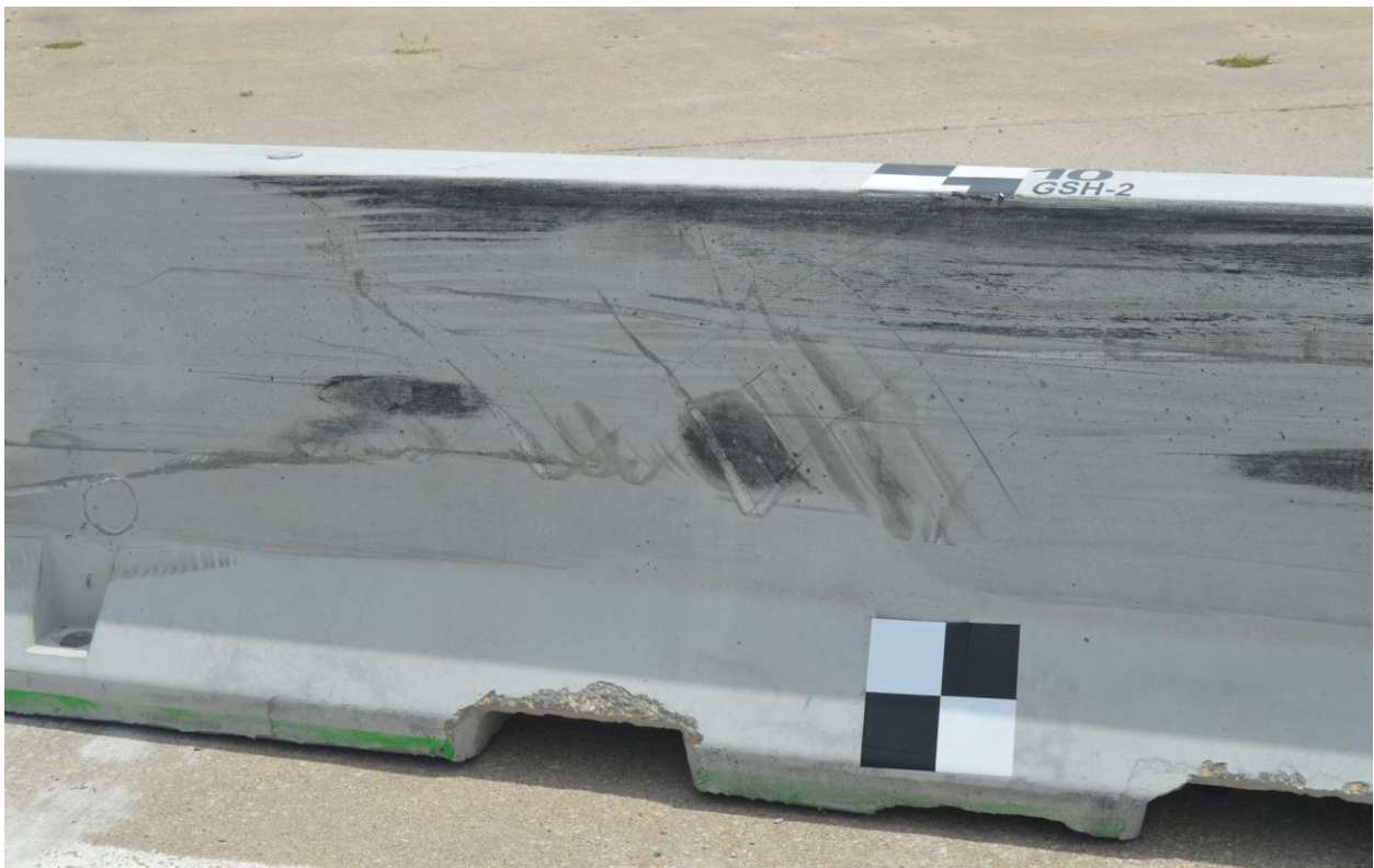
Figure 77. Barrier No. 10 Damage, Test No. GSH-2
