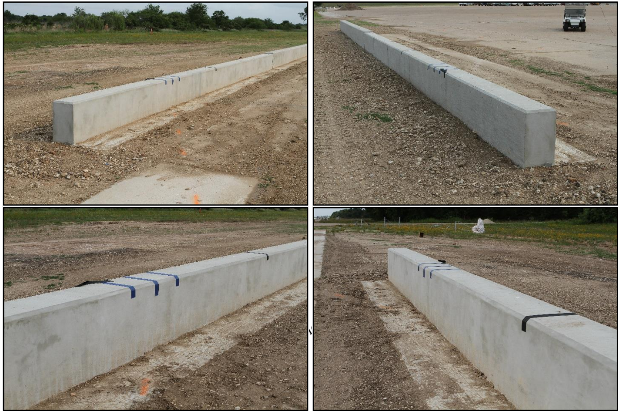
Figure 3.2 Permanent Low-Profile Barrier prior to Testing.
