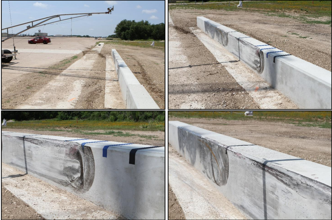
Figure 6.3 Permanent Low-Profile Barrier after Test 616151-01-2.
