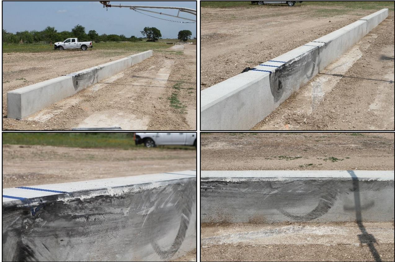
Figure 7.3 Permanent Low-Profile Barrier after Test 616151-01-1.
