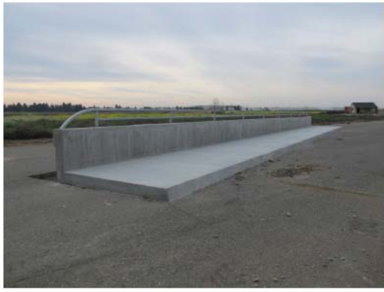
Figure 2-6 – Type 732SW with the steel handrail in place
