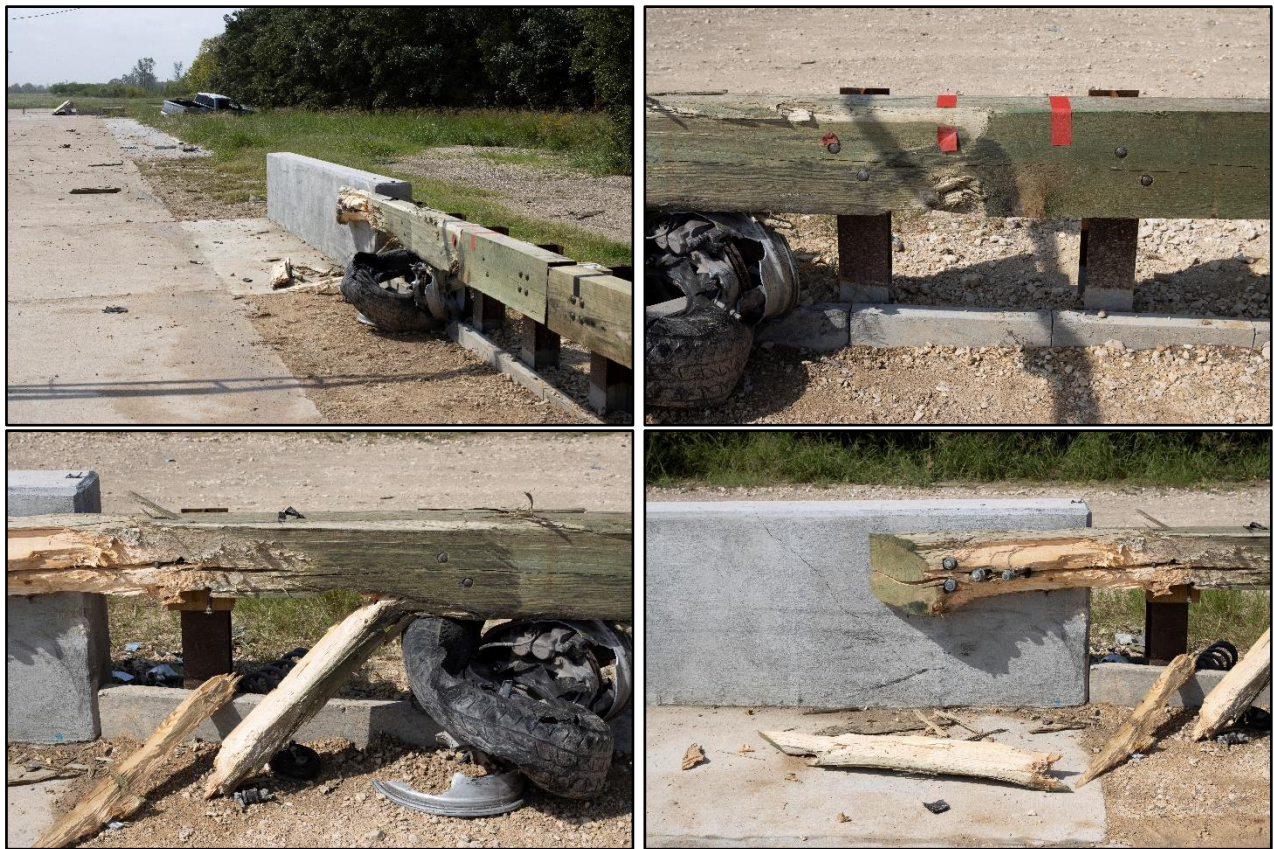
Figure 6.11. Transition after Test No. 612061-06-1.
