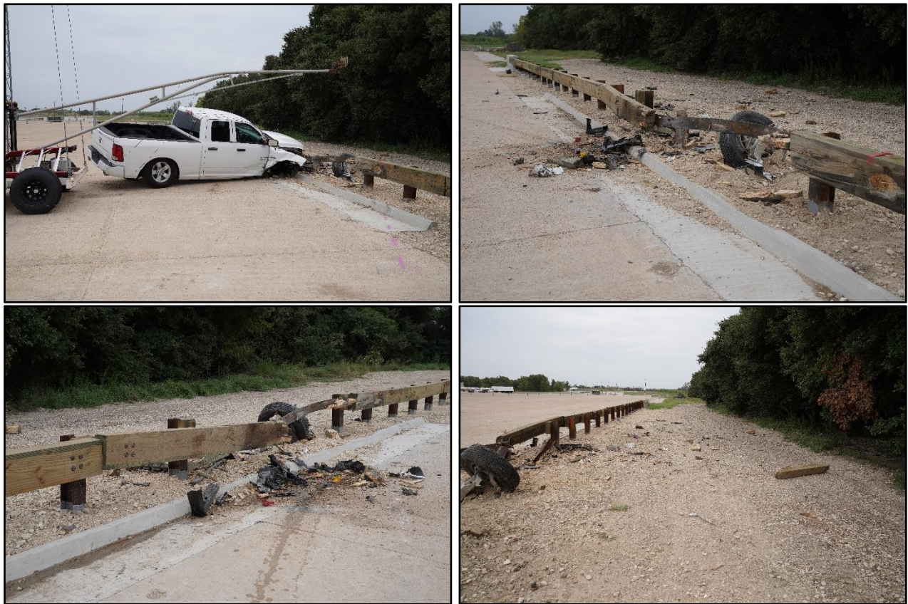
Figure 5.5. Modified Merritt Parkway Guiderail after Test No. 612061-02-1A.
