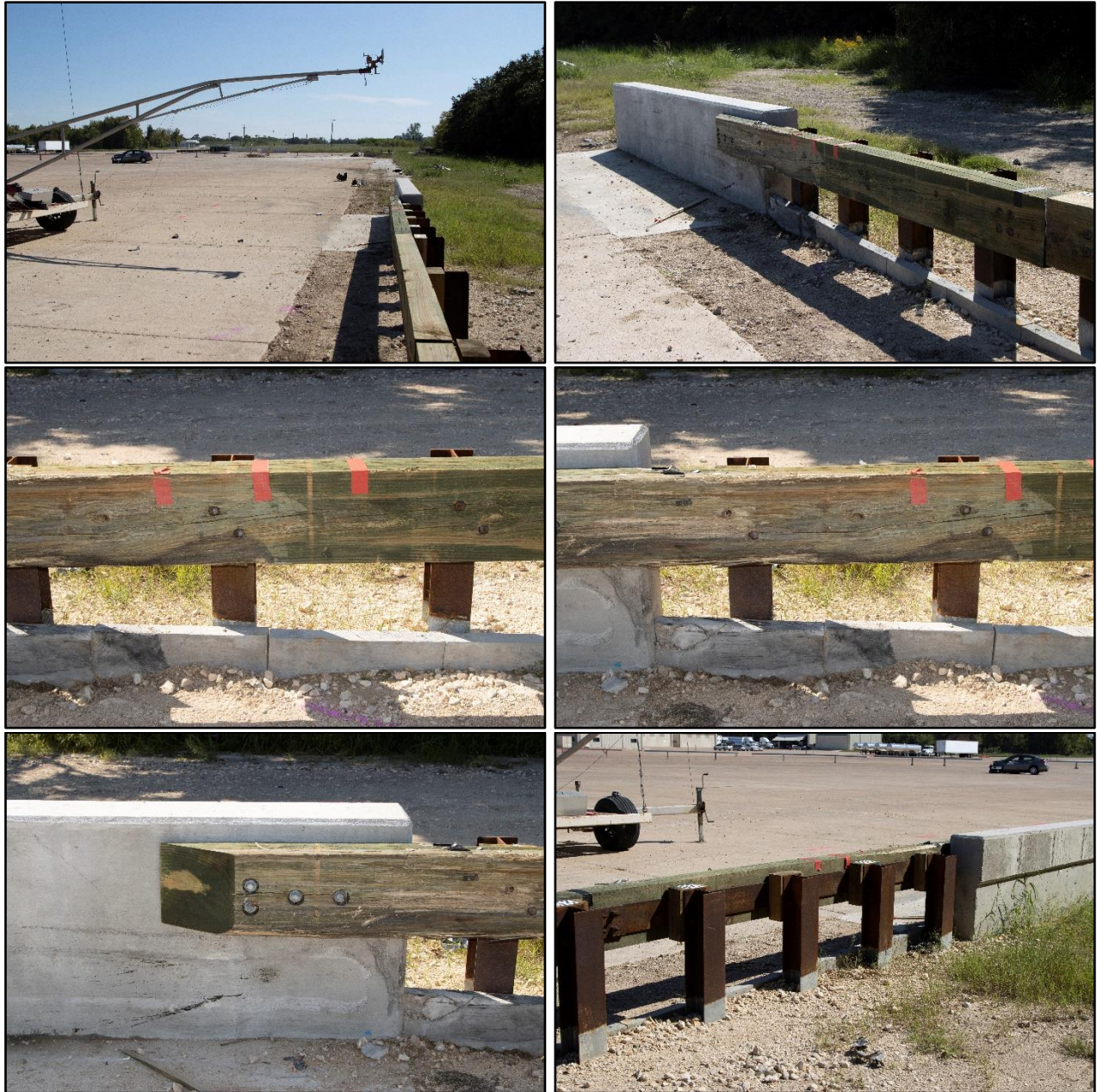
Figure 6.5. Transition after Test No. 612061-07-1.
