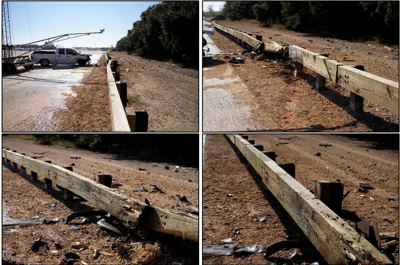
Figure 4.5. Merritt Parkway Guiderail after Test No. 612061-02-1.
