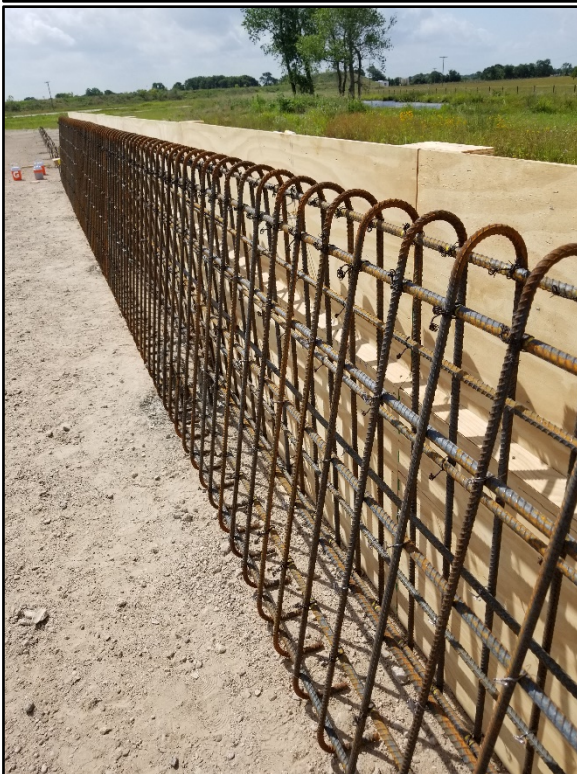
Figure 3.2. SSCB with the Drilled Shaft Foundation Construction.
