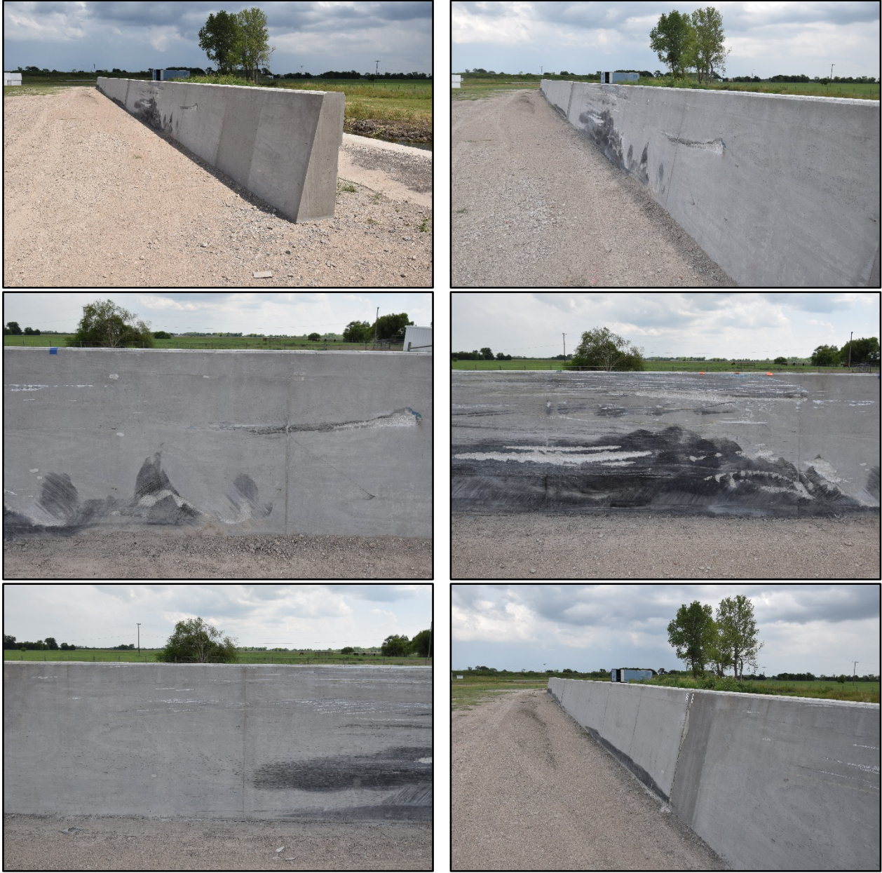
Figure 6.3. SSCB after Test No. 469489-01-3.
