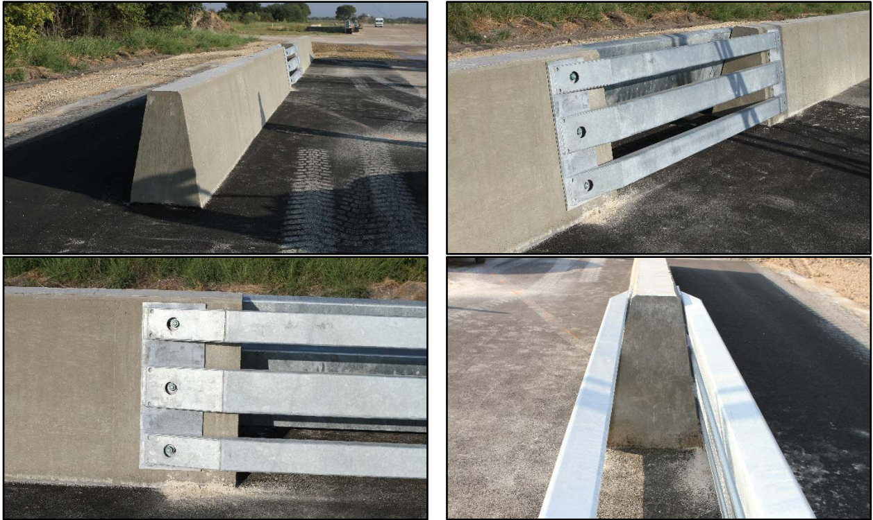
Figure 1. Barrier Gap Design before Test No. 610461-2.
