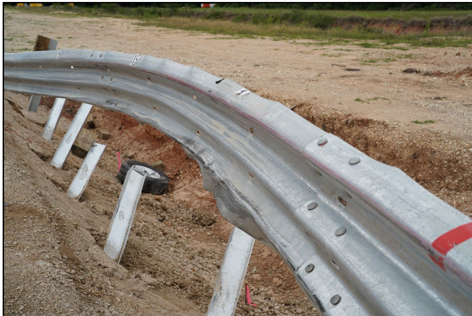
Figure 7.6. Guardrail System on 1:1 Slope at Impact Location after Test 617771-01-2.
