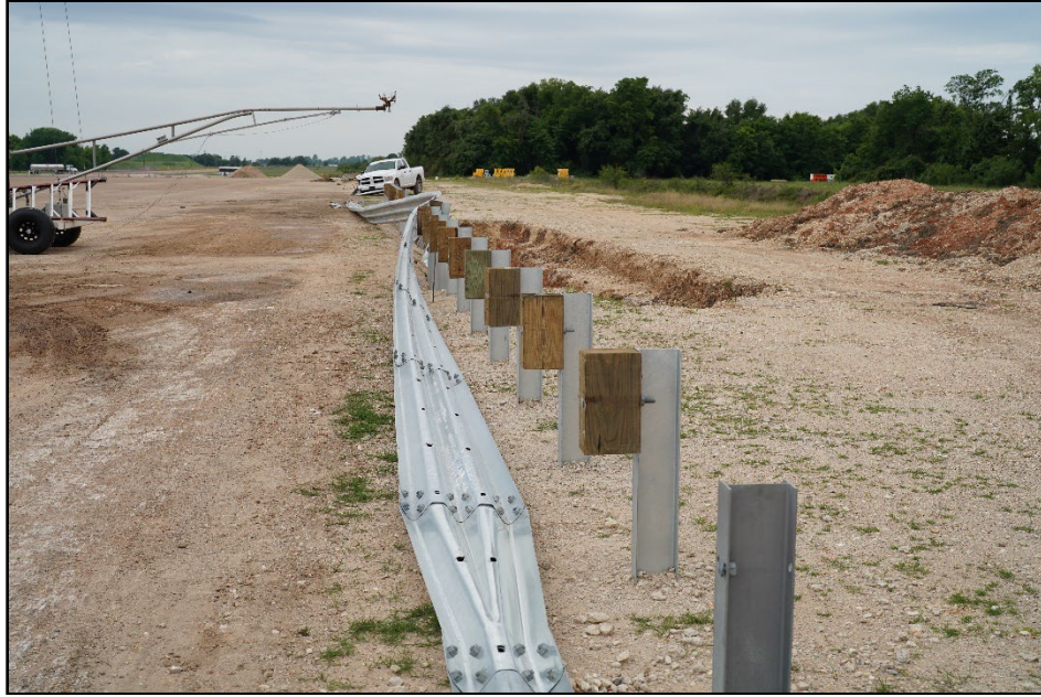
Figure 7.5. Overall View of the Guardrail System on 1:1 Slope after Test 617771-01-2.
