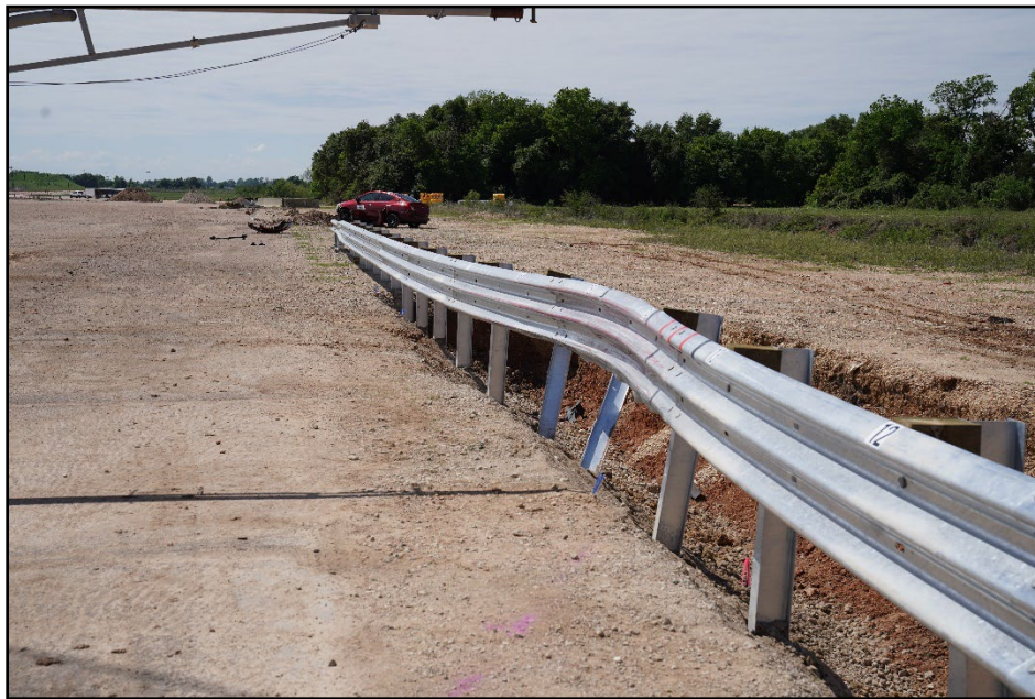
Figure 6.5. Guardrail System on 1:1 Slope at Impact Location after Test 617771-01-1.
