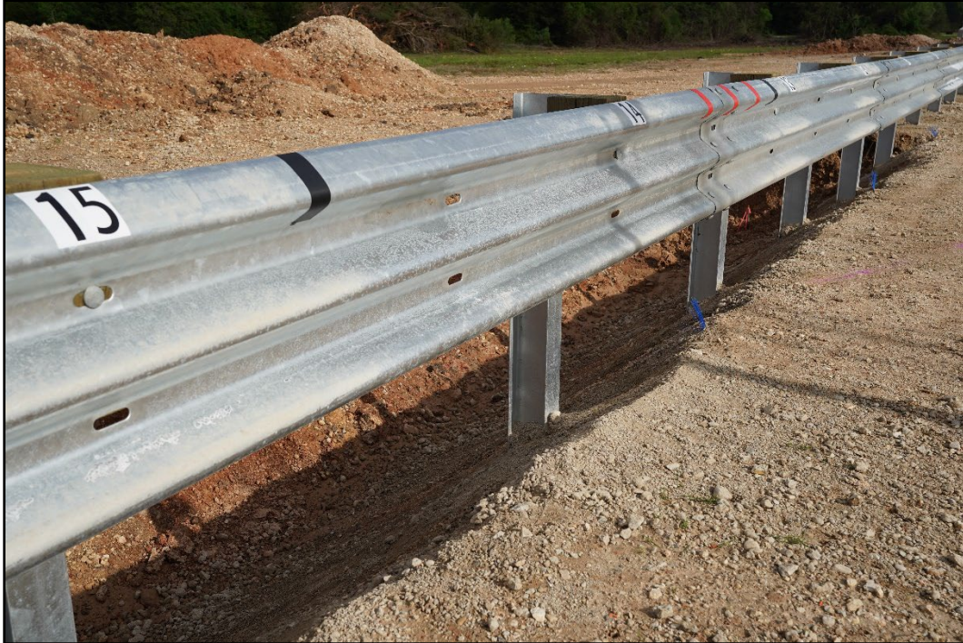
Figure 3.4. Guardrail System on 1:1 Slope at Impact Prior to Testing.
