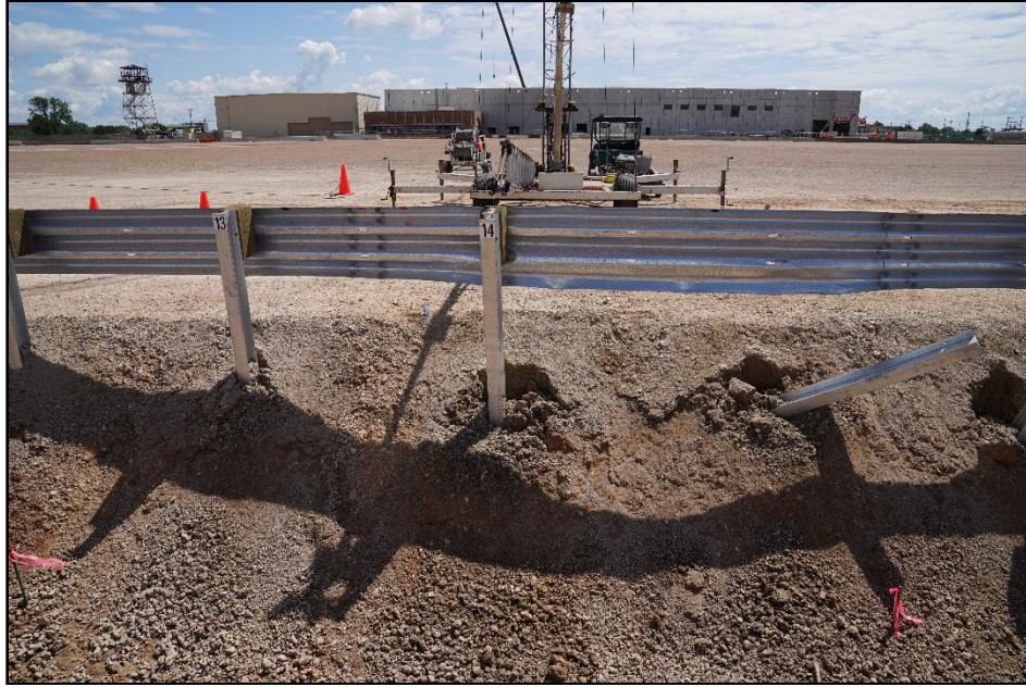
Figure 6.6. Guardrail System on 1:1 Slope from the Field Side after Test 617771-01-1.
