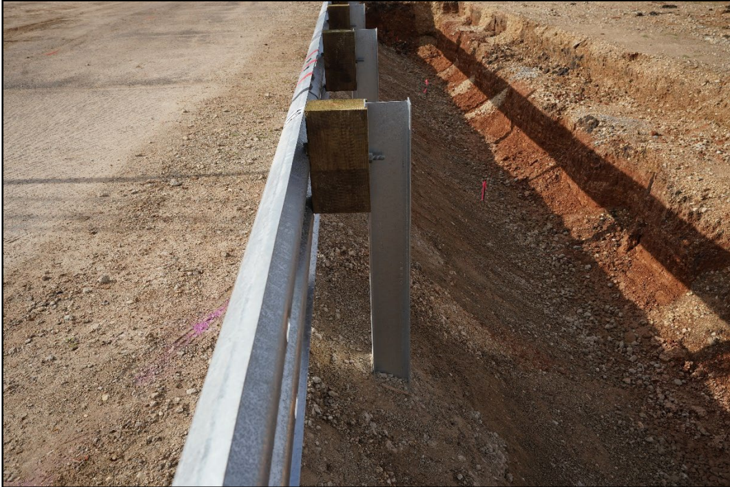
Figure 3.6. Detail of Posts in Guardrail System on 1:1 Slope Prior to Testing.
