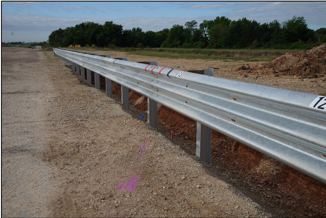
Figure 3.2. Overall View of the Guardrail System on 1:1 Slope Prior to Testing.
