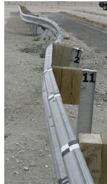
(c) Installation After Test
