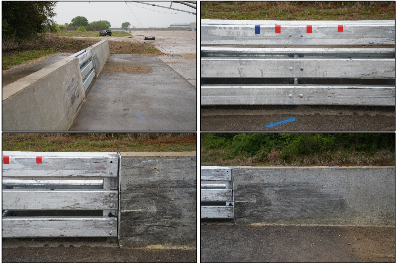
Figure 5.3. Redesigned Barrier Gap Rail after Test No. 610461-01-3.
