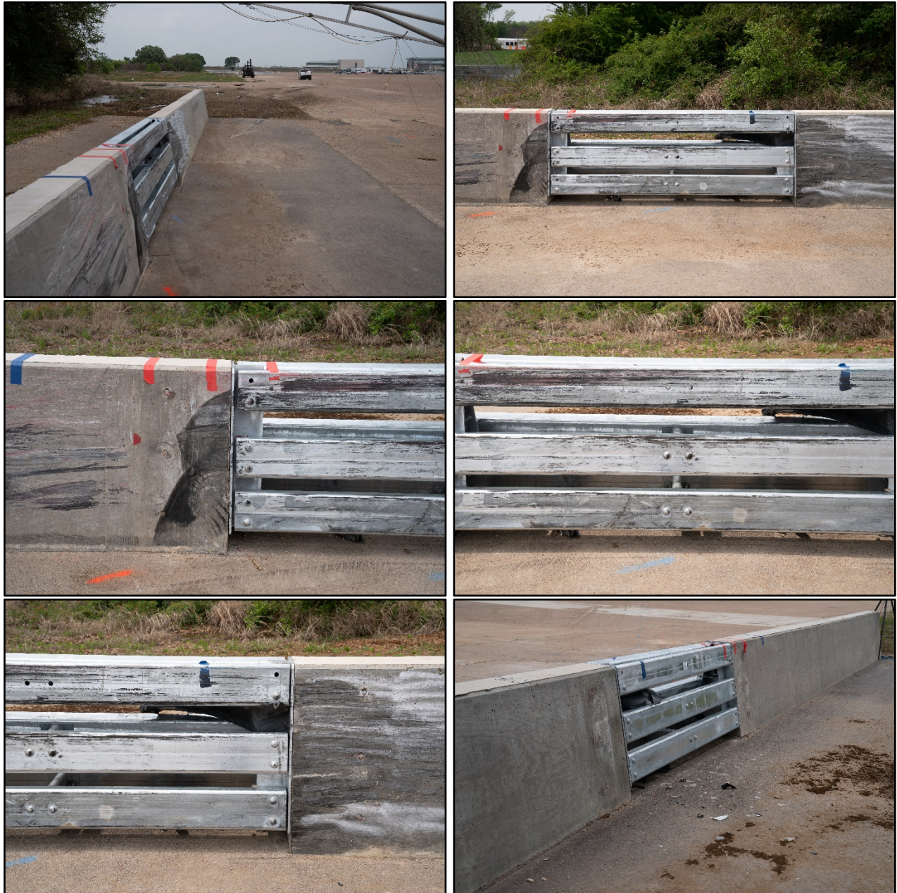
Figure 6.3. Redesigned Barrier Gap Rail after Test No. 610461-01-4.
