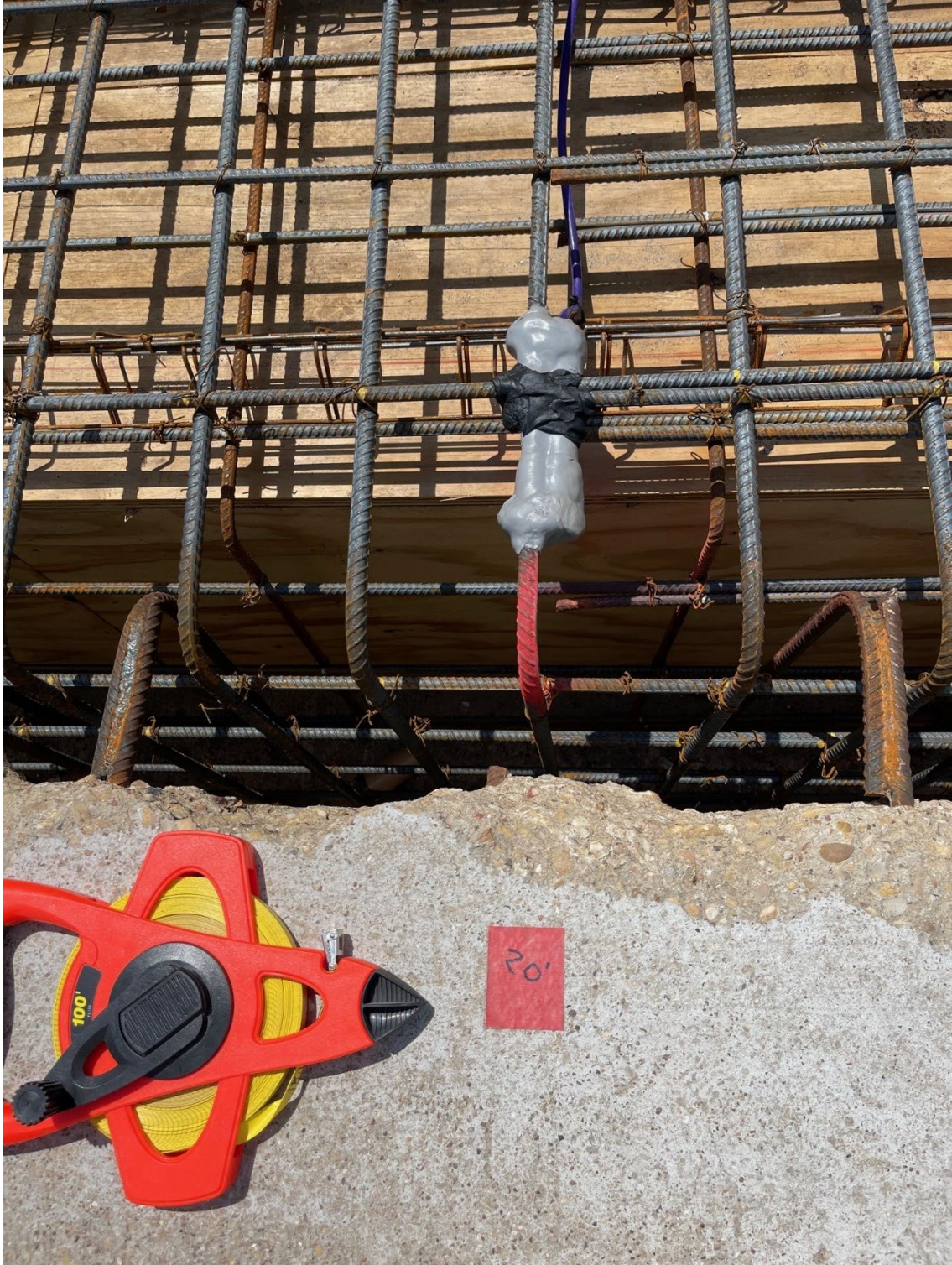
Figure 7 – Layout of Strain Gauge
