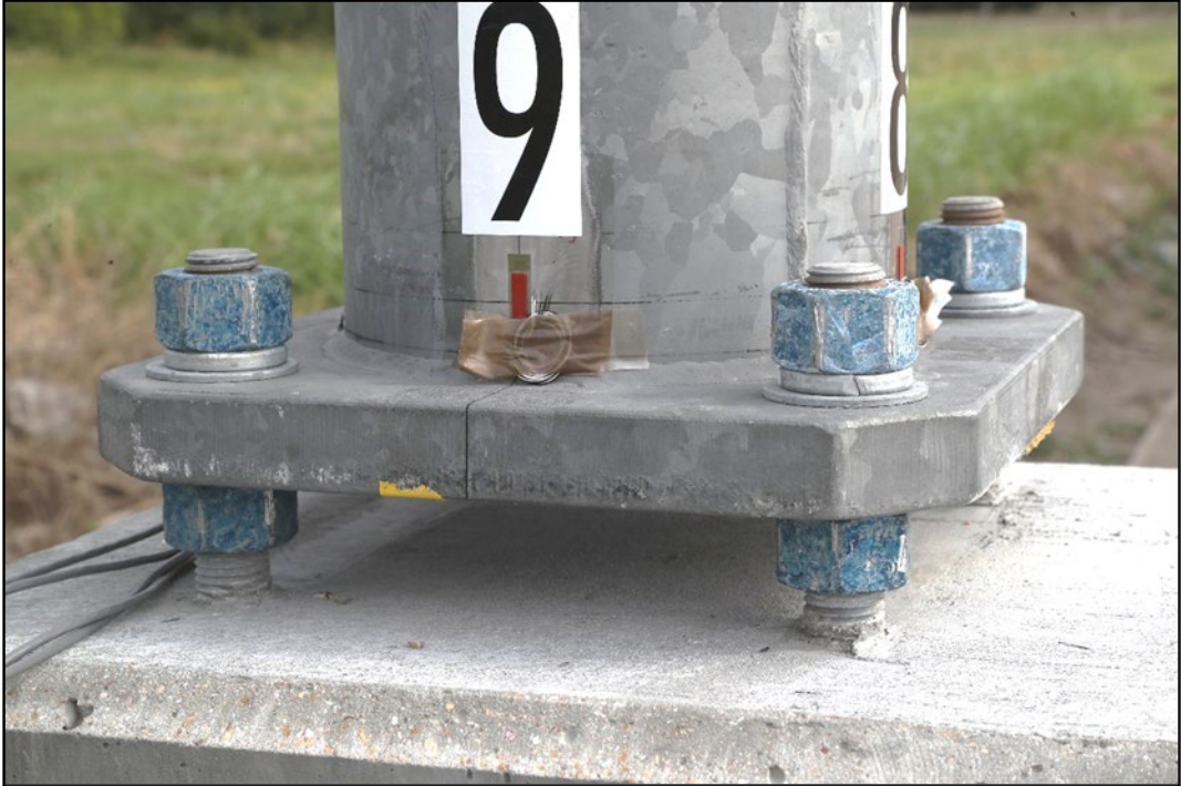
Figure 5 – Photos of Strain Gauges on Light Pole
