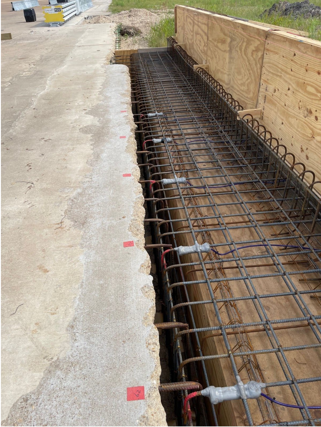
Figure 6 – Layout of Strain Gauges
