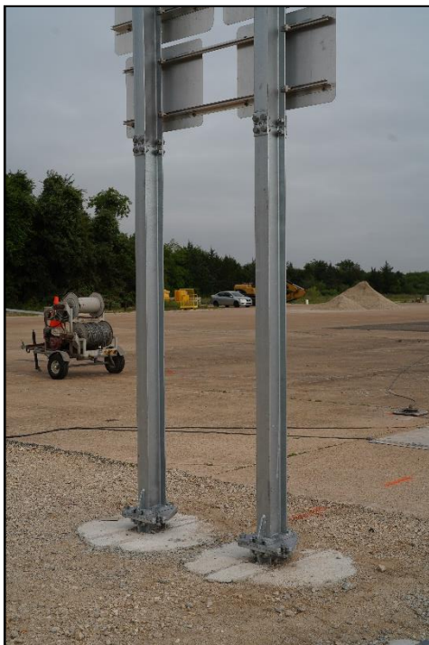
Figure 4-5. Back Side of the Route Marker Assembly with Large Sign Supports prior to Testing.
