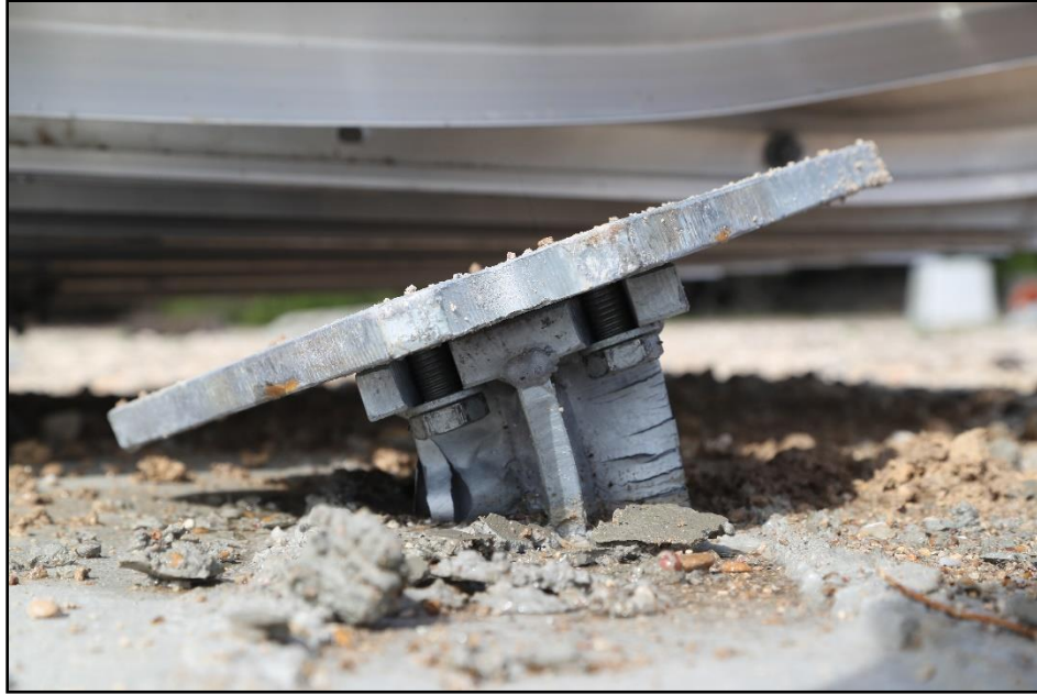
Figure 12-6. Footer for the Guide Sign with Large Sign Supports after Test 616401-01-8.
