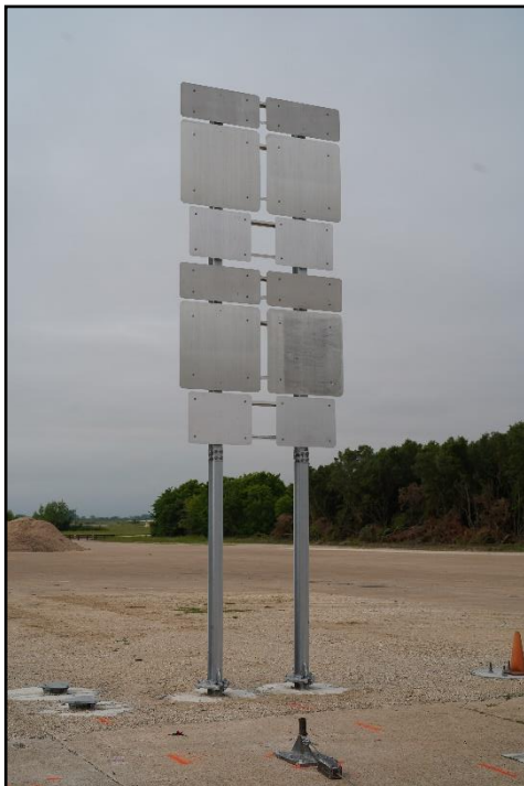
Figure 4-4. Impact Side of the Route Marker Assembly with Large Sign Supports prior to Testing.
