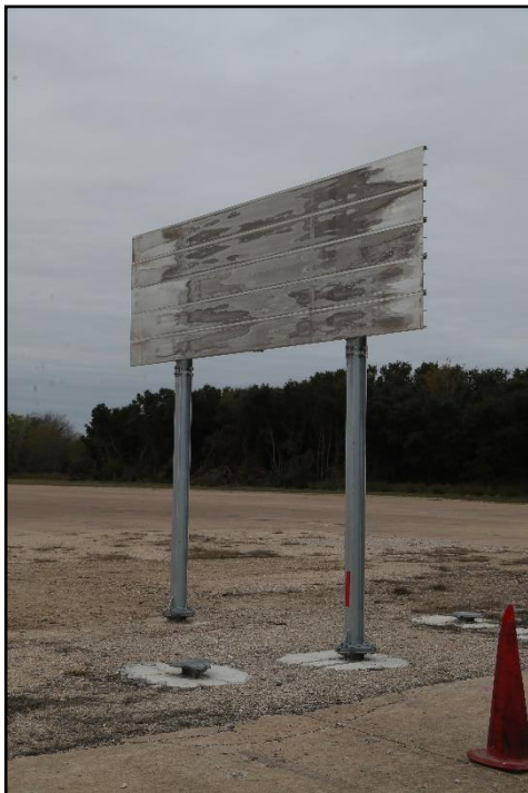
Figure 4-19. Impact Side of the Guide Sign with Large Sign Supports prior to Test 616401-01-4.
