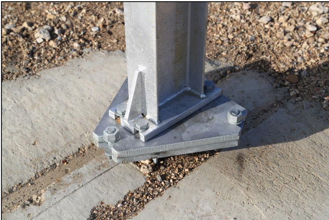
Figure 4-27. Slip Base on the Guide Sign with Large Sign Supports prior to Test 616401-01-8.
