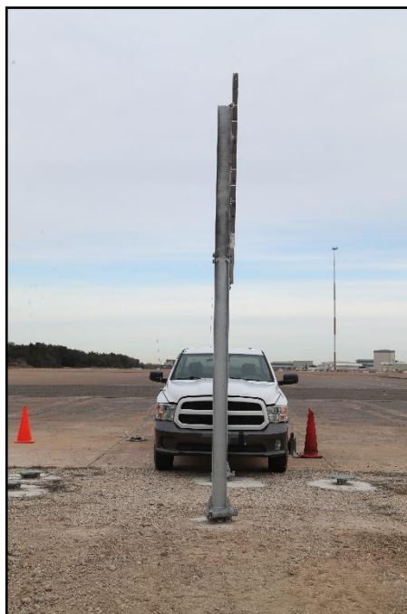
Figure 11-2. Guide Sign with Large Sign Supports /Test Vehicle Impact Location 616401-01-4.
