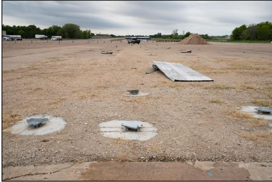
Figure 10-5. Guide Sign with Large Sign Supports at Impact Location after Test 616401-01-9.
